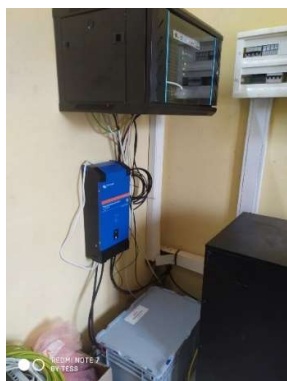
Figure 6: A solar powered VHF repeater site, with Power inverter connected to batteries, solar panels feeding SCS equipment in the rack
