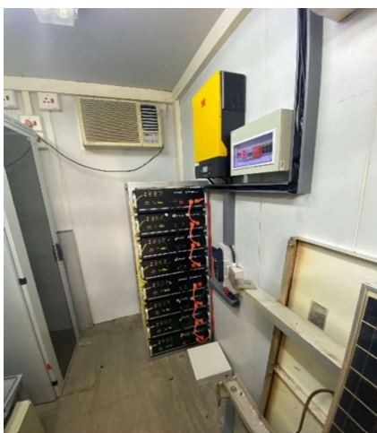
Figure 10: Solar panel inverter with UPS and batteries for a VHF repeater site
