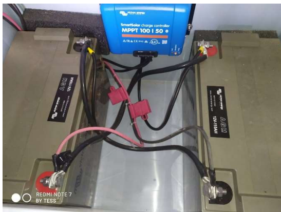
Figure 8: Battery connections to a solar panel controller
